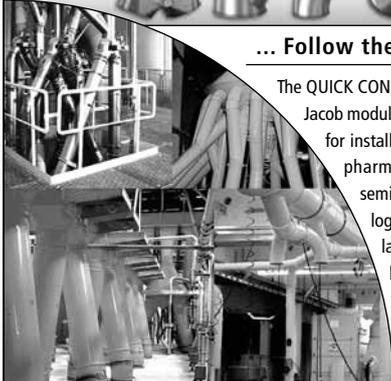
The QUICK CONNECT® pull-ring makes the acclaimed Jacob modular pipe system even more economical for installation. In new plants for animal feed, pharmaceuticals, chemicals, food, glass, semiconductors or environmental technology as well as for upgrading existing layouts user-friendly system installation becomes precise and easy due to the great versatility of mass-produced pipe components.
